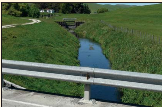
Lake Poukawa Control Gates
